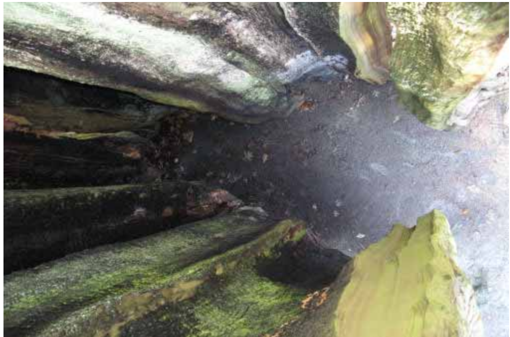
Photo 6: Looking down centre of Hollow Tree at weakened "C" shaped cross section
