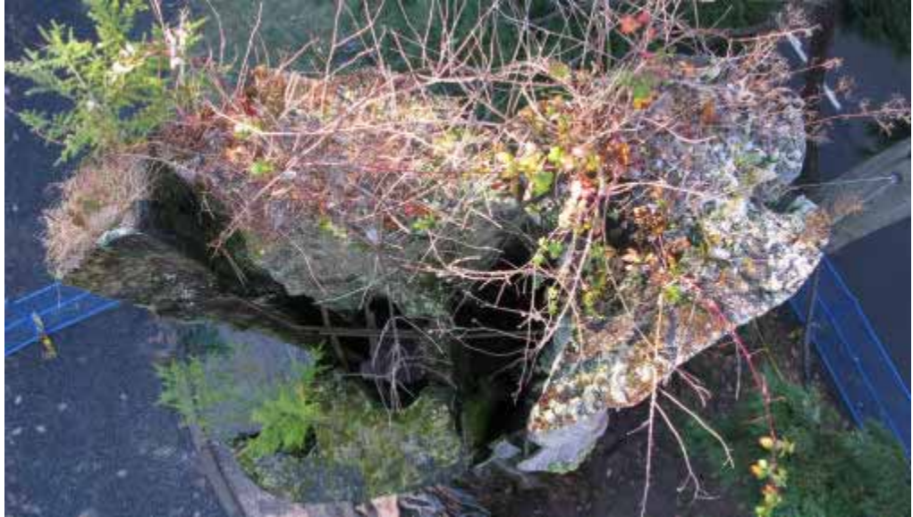
Photo 7: Top of trunk showing decay of exposed end grain
